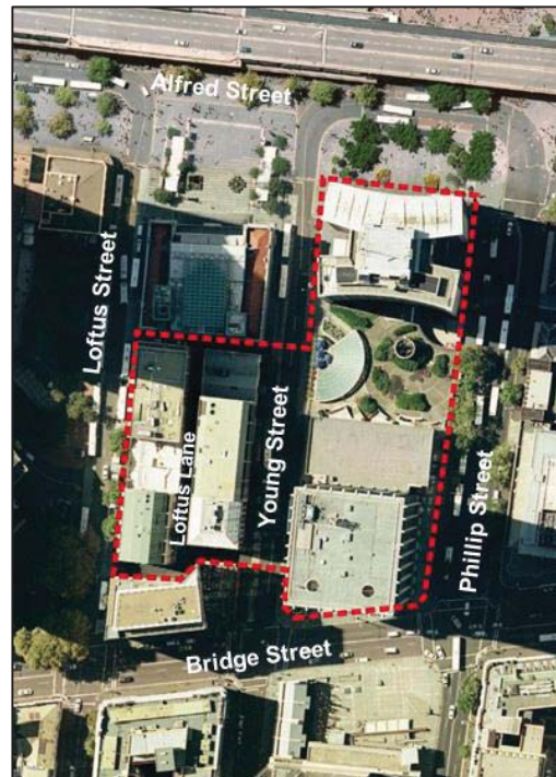
Figure 2: Aerial photograph of subject site
