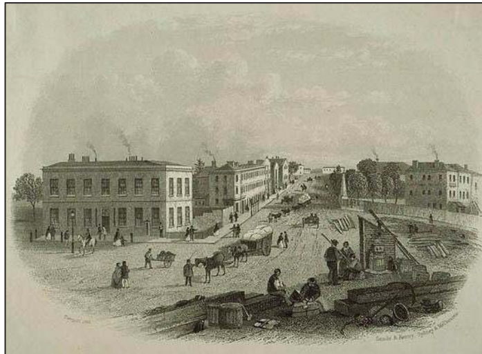
Figure 13: c. 1862 engraving showing Customs House and buildings along Loftus Street
