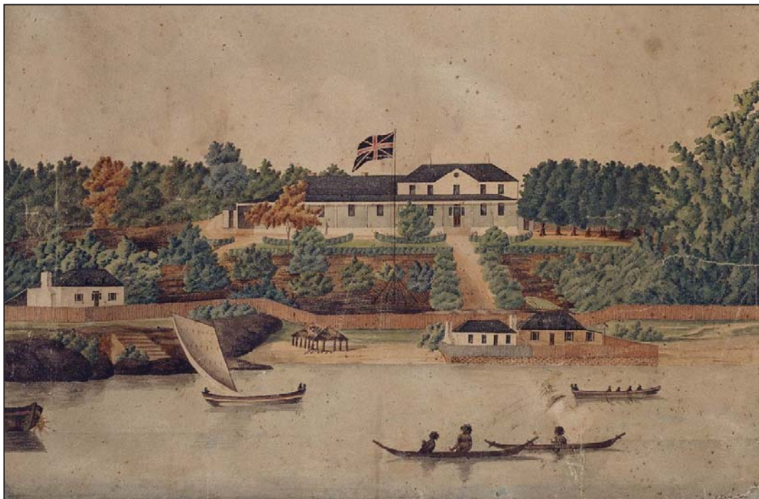
Figure 9: First Government House c. 1807
